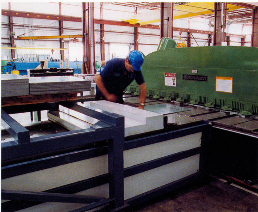
The shear installation mates a Canrack/PMI feeder with a 12-ft. Cincinnati mechanical shear. The shear feeder advances sheets at 1100 in./min. for all weights, and positions to an accuracy of \pm 0.005 in.
